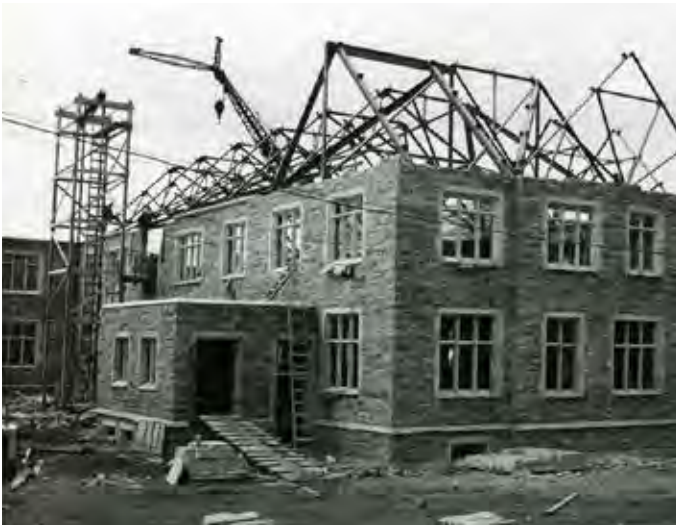
USask, University Archives & Special Collections, Photograph Collection, A-2191 "Memorial Union Building – Construction", 1954. Photography: Saskatoon StarPhoenix
